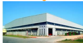
Building CCTV System
